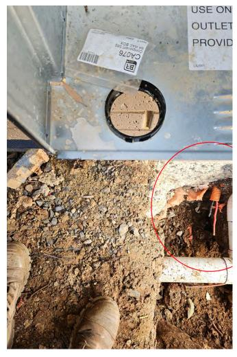
Site unacceptable Concrete overspill and storm water pipes in the way
