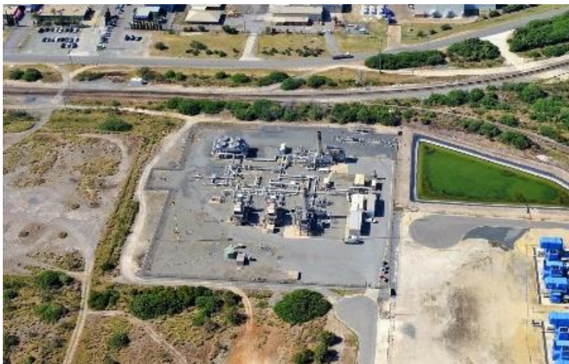
Figure 8.3: Aerial view of Compressor Station 10
