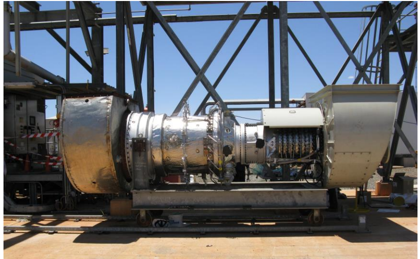
Figure 7.7.2: Turbine exchange, Compressor Station 2, Unit 3, September 2018
